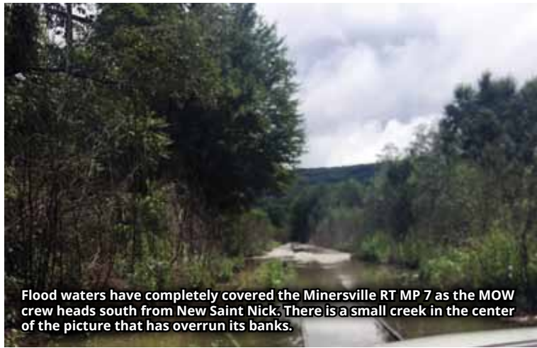
Washouts like this one on the M&S Branch are common with the amount of rainfall and water we have had this past year. Once each washout is identified, MOW gangs are sent out to install a pipe and restore the track structure.
