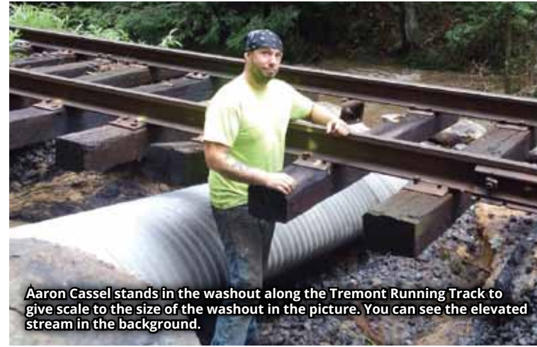
The shoulder along the Tremont Running Track was washed away as well as our ditch along the tracks filled with material. Most of the ballast that was in our track was pushed into our ditches. This type of damage was seen over miles of track.
