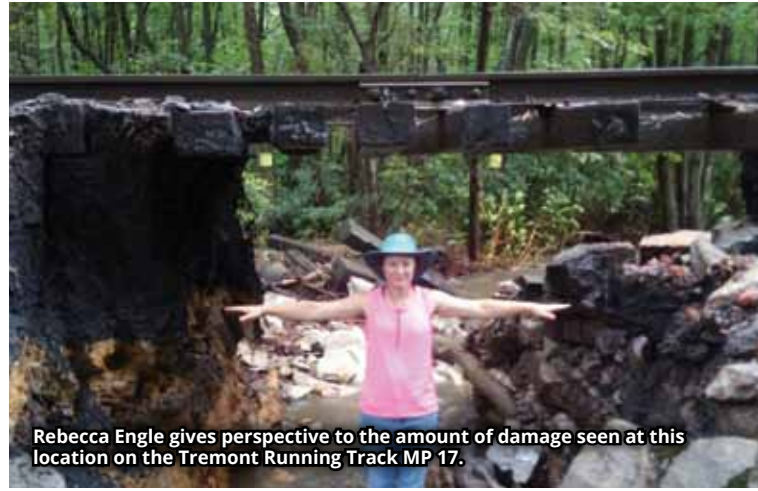
An additional pipe was installed on the Tremont Branch to assist with the large volumes of water experienced during the flooding. This location was repaired the previous day and a new pipe installed. The additional flooding overnight all but erased any work from the previous day.
