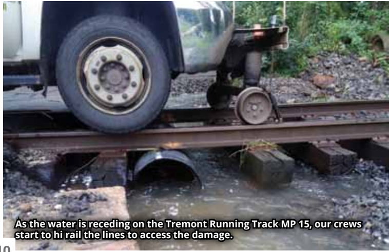
This type of washout along the Tremont Branch north of MP 14 was a result of the large volumes of water heading to the small creek that paralleled our tracks.
