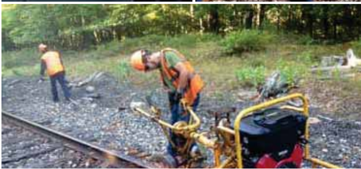
One piece of equipment used in the crop and weld process used by GWPeoples to eliminate joints on #2 track. Frank Sebelin takes the picture as he keeps the gang working.
