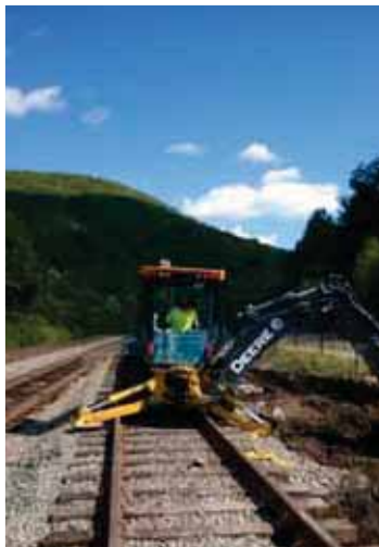
Brendle Stufflet finishes backfilling around the new cantilever base at MP 124.77 Coal and continues to clean up the access fill along the track.
