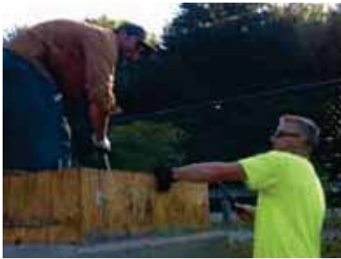
Dave Hutton (Signal Department) assisting with Mario DeMarco (MOW) to remove forms on the cantilever base at MP 124.77 Coal.
