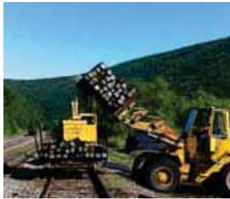
W.E. Yoder loads up the new ties being laid out along the Lehighton Branch as the gang begins a tie replacement project.
