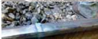
One more step is needed to finish off this newly flash butt welded rail.
