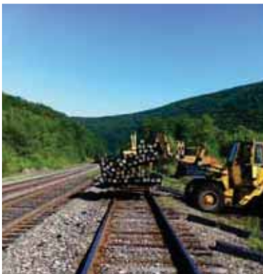
W.E. Yoder with Matt Minnich work on laying out ties on the Lehighton Branch MP 121
