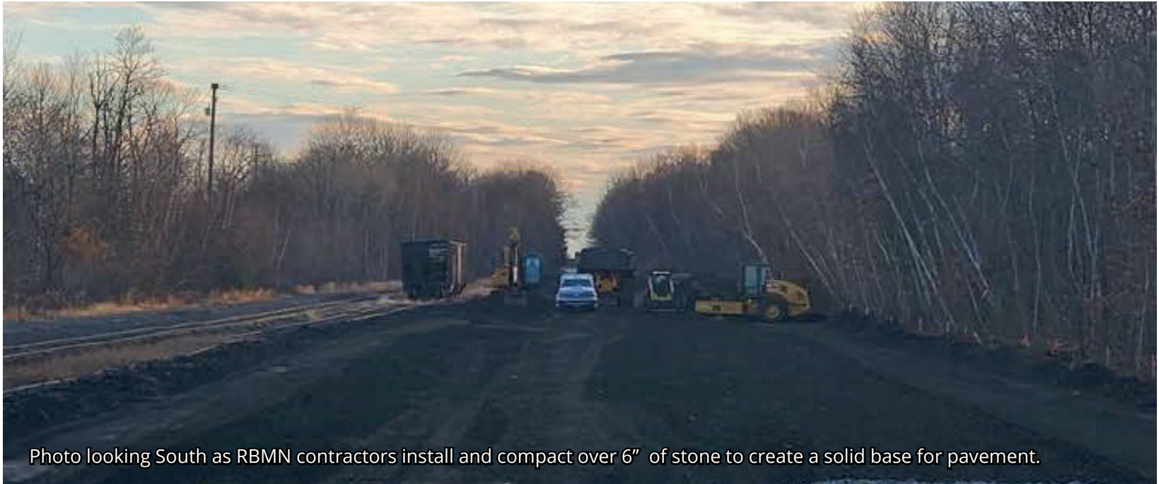
RBMN contractors and equipment hard at work removing trees/brush and beginning the process of backfilling and leveling ground at the Locust Summit site.
