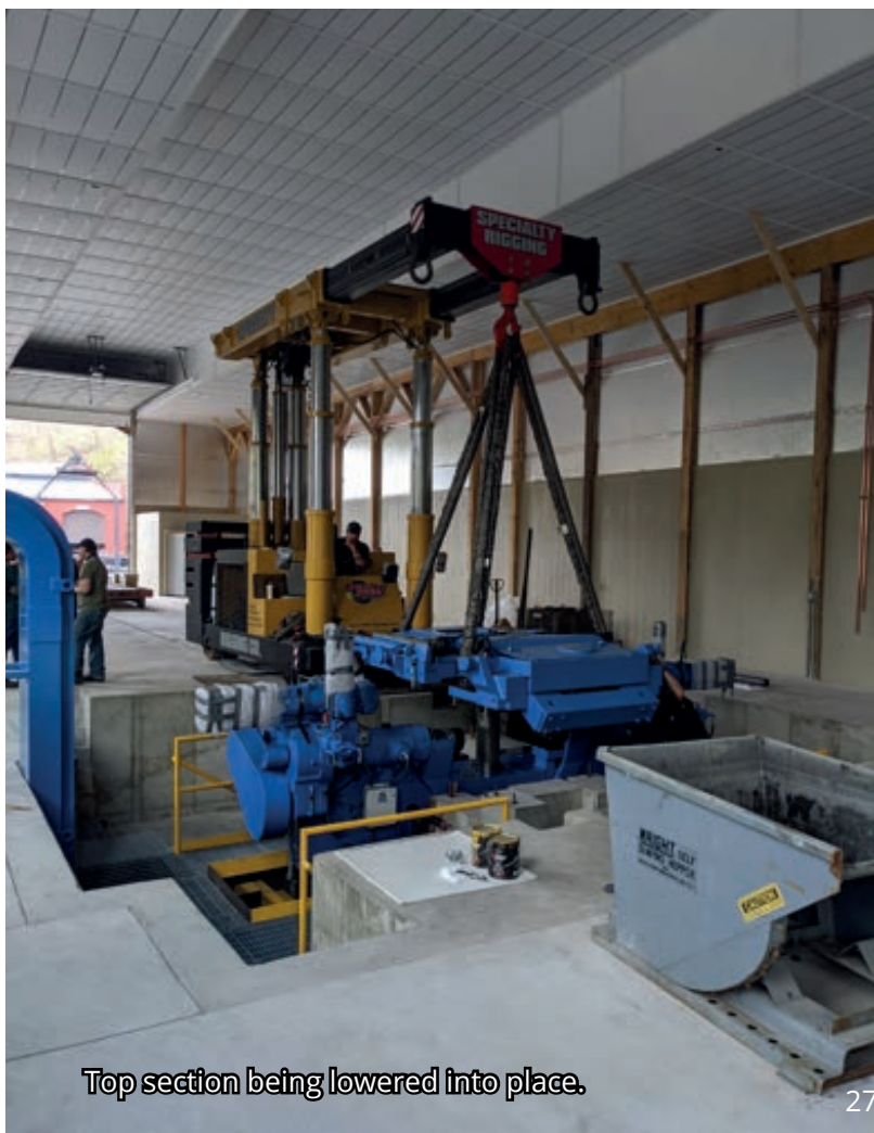
C-frame awaiting the placement of the top section.
