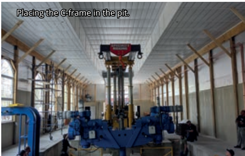
Tri-lifter getting C-frame in place.
