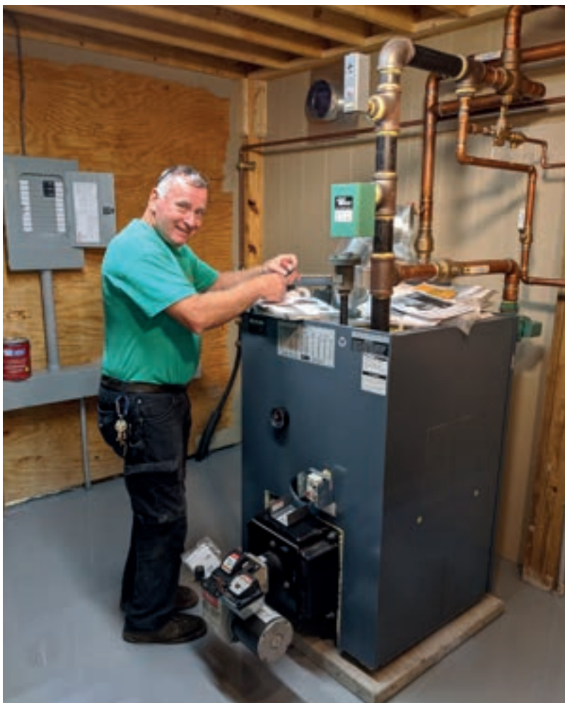
Bill Keim works on the boiler for the floor heat system.
