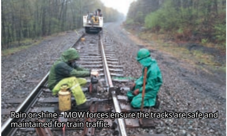
Corey Hamm performing a thermite weld at ML MP 116.8.
