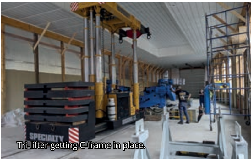
Placing the C-frame in the pit.
