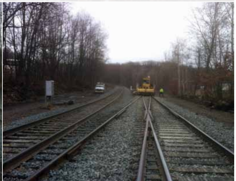
North facing view, ballast regulator providing final touches. Photo by Duane Engle.
