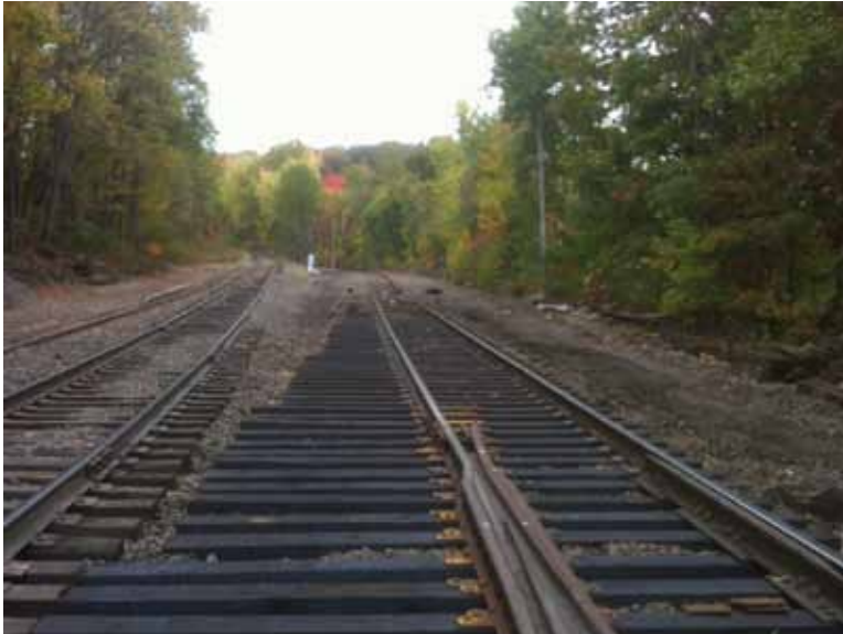
Multiple switch timbers installed, facing north. Photo by Duane Engle.
