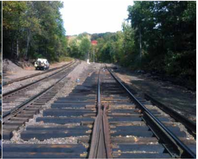
First of two frogs installed, facing north. Photo by Duane Engle.
