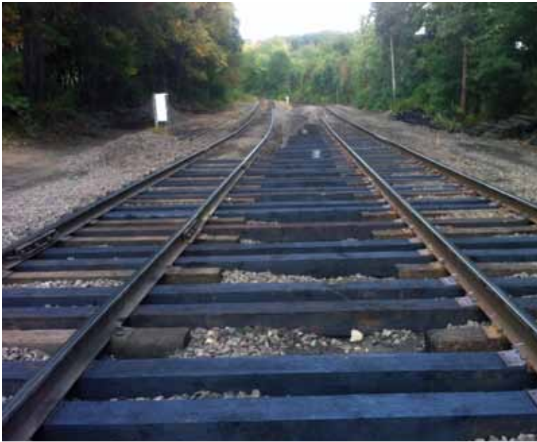
Multiple switch timbers installed, facing north. Photo by Duane Engle.
