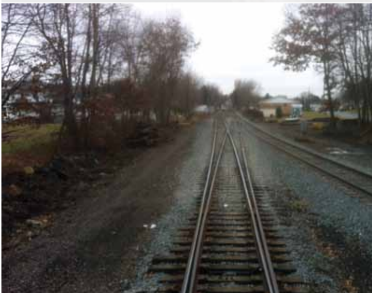
South facing view of finished product. Photo by Duane Engle.
