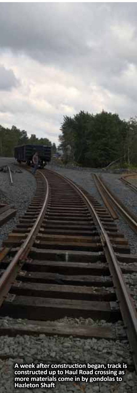
The track subgrade is prepared as materials and tools begin to be unloaded in preparation for the construction of a siding for service to Hazleton Shaft.
