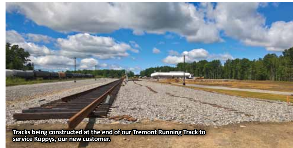
Prepared subgrade is ready for track construction as materials are laid out along the future track.
