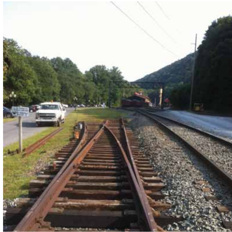
Addition of second switch at MP 78.35 for another track off the new Car Shop Lead in Port Clinton yard.
