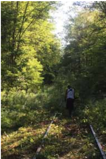
Greenwood Running track covered by thick brush and weeds. Prior to clearing this section clean of vegetation, the ROW was only recognizable by break in the tree canopy above.
