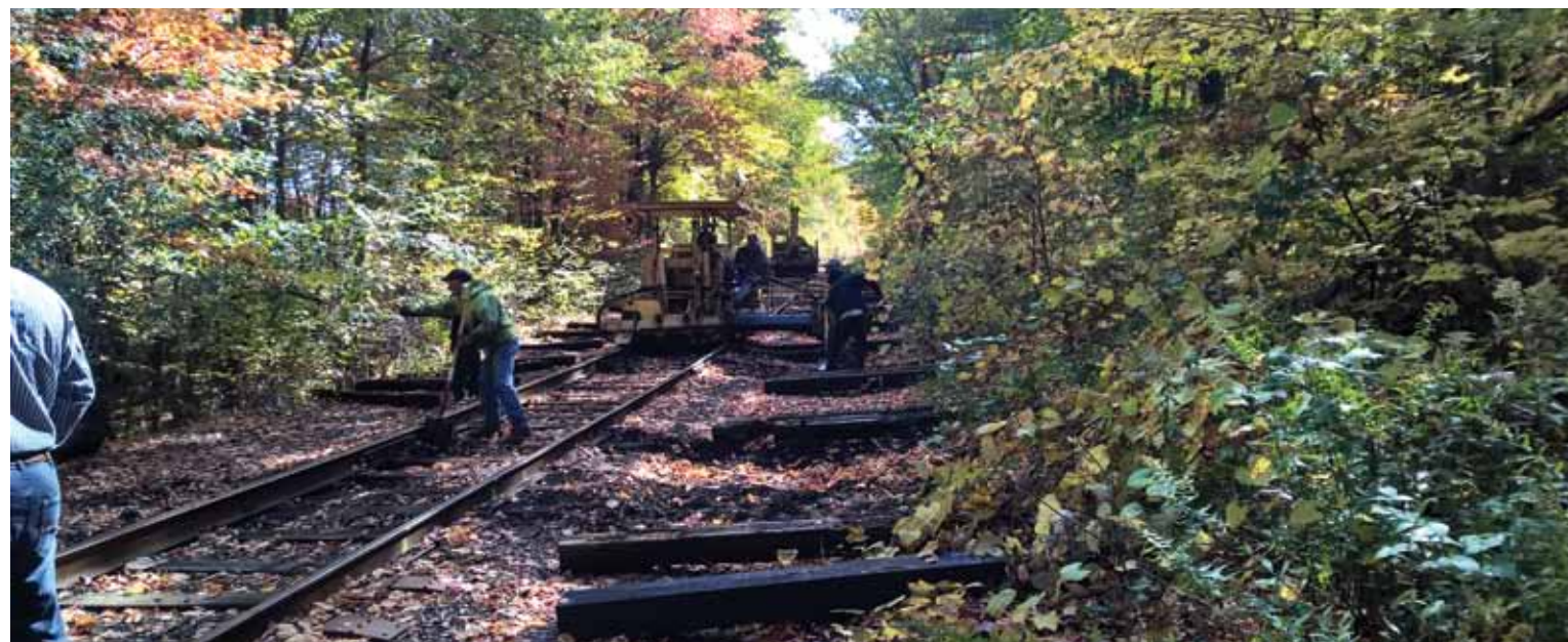
W. E. Yoder tie gang installing ties on Hazleton Line MP 106.7.
