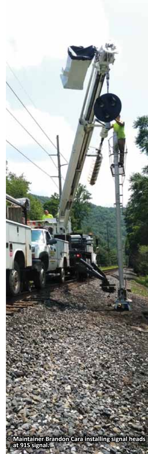
Maintainer Graham Hantz installing the signal heads for northbound moves out of Clint Interlocking.
