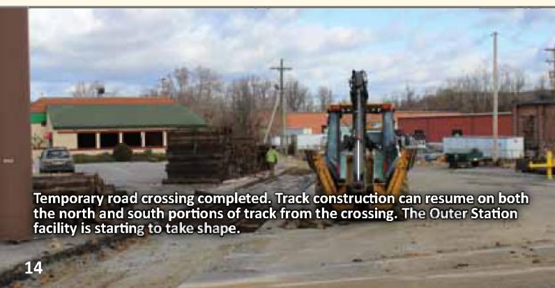
Ties are laid out with tie plates installed to start the rail installation at Outer Station. Stacks of ties are prepped and ready for the remaining track construction to this new facility.
