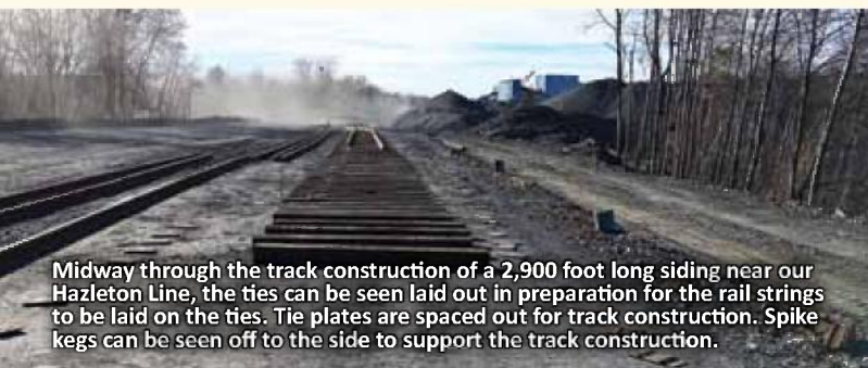
To accelerate the track construction, rail strings in 156 foot lengths were brought in and laid out next to the track. These strings eliminate additional joints required on standard thirty nine foot rail lengths.
