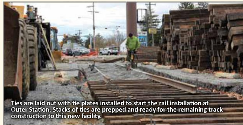
First step in the construction of track is to make a crossing to access either side of the new track construction through the parking lot. Ben Cole is pictured running a hydraulic hand tamper to level the rail to the parking lot surface.
