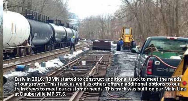
Track construction at MP 68 on our Main Line just outside Dauberville is well under way. Once this project was finished, RBMN had an additional mile of track for operational use by train crews.
