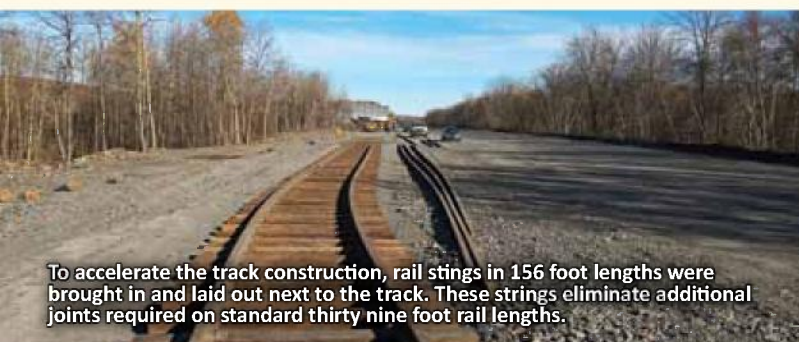
Another new siding constructed to serve a customer near our Hazleton Line. Once completed the siding was 2,900 feet long.
