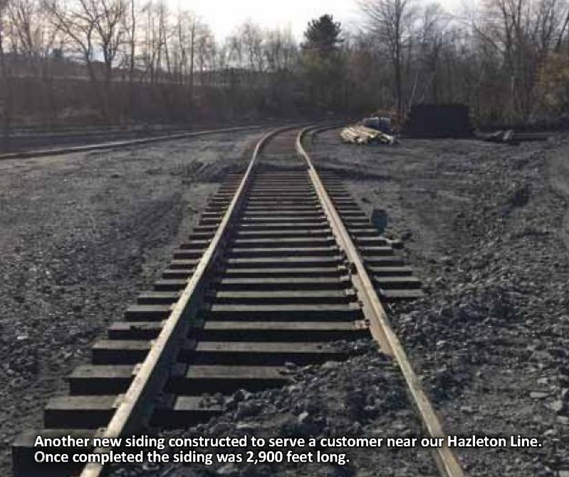
Skeleton track constructed to serve another customer near our Hazleton Line. New subgrade was built and made ready for track construction.
