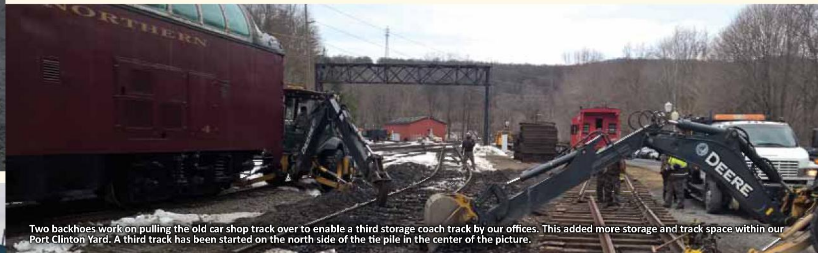
Port Clinton Yard also received some new track construction for more storage space. The car shop lead was added to a new track constructed along the driveway to make improvements to passenger loading in Port Clinton Yard. The track is also utilized every day to shift cars in and out of the Car Shop.
