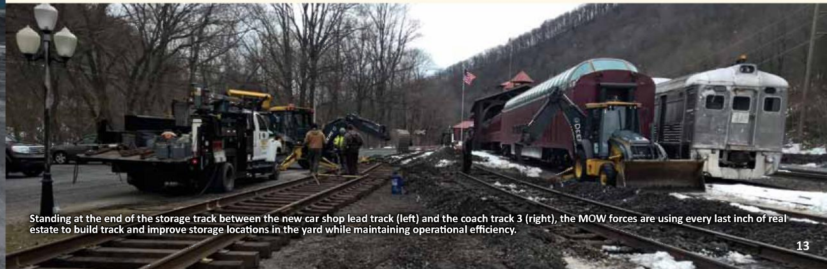
Two backhoes work on pulling the old car shop track over to enable a third storage coach track by our offices. This added more storage and track space within our Port Clinton Yard. A third track has been started on the north side of the tie pile in the center of the picture.
