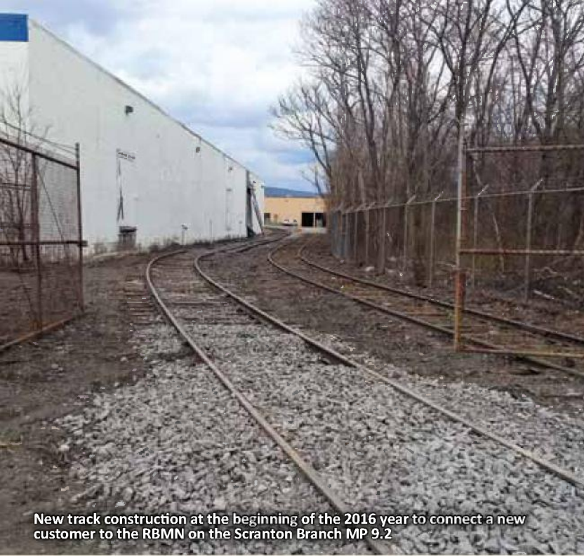
New switch installed on Scranton Branch MP 9.2 to welcome a new customer to RBMN. Switch and siding rehabilitated to bring service back to building that used rail service in the past.
