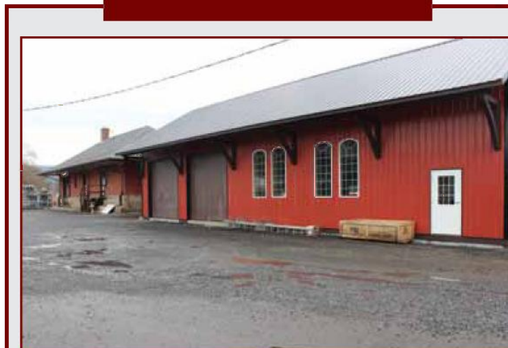
Newly constructed Cressona Signal Warehouse.
