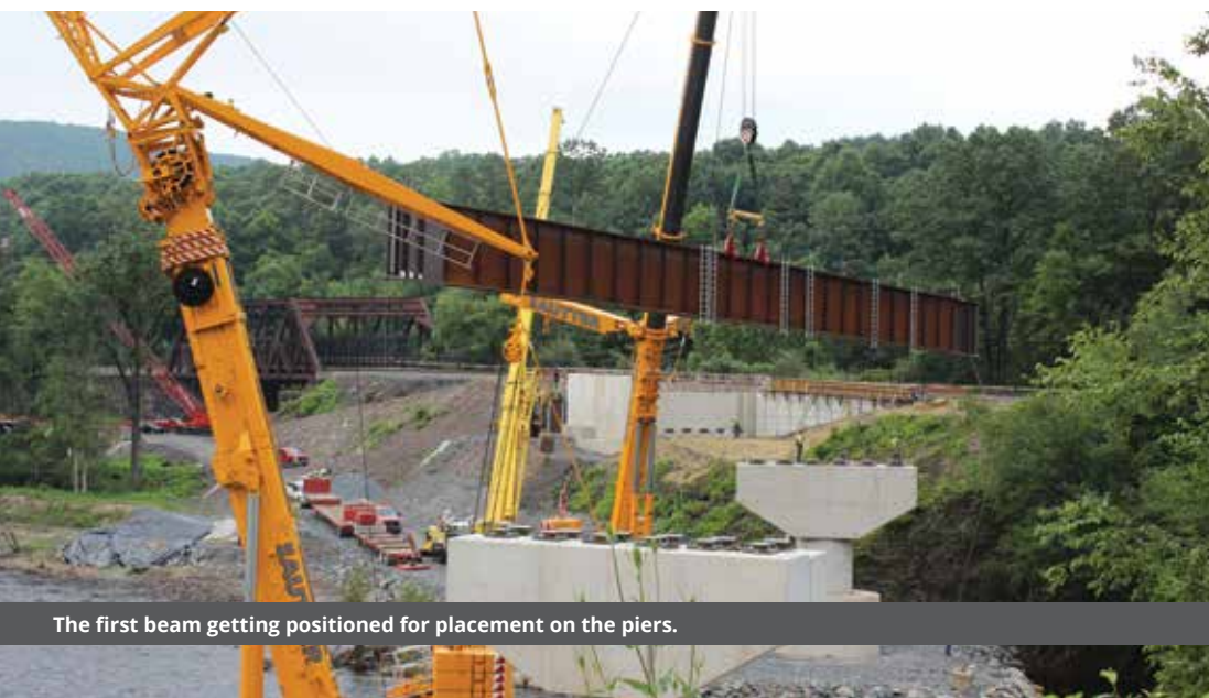
Early morning July 11, the first three beams have arrived and are getting prepped for placement on the bridge piers.
