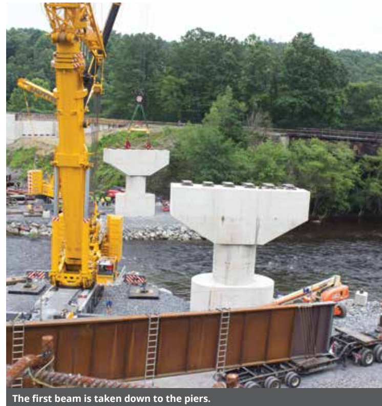
The first beam is taken down to the piers.
