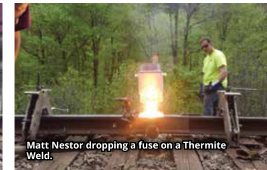
Matt Nestor heating up a Thermite Weld at MP 144.
