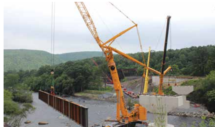
The massive beam is lifted over the Lehigh River.
