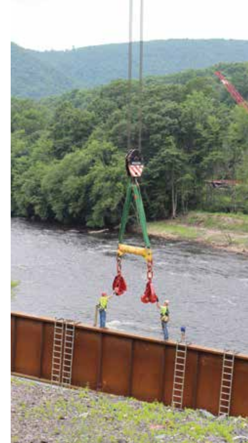
The first beam is attached to the crane for lift off.
