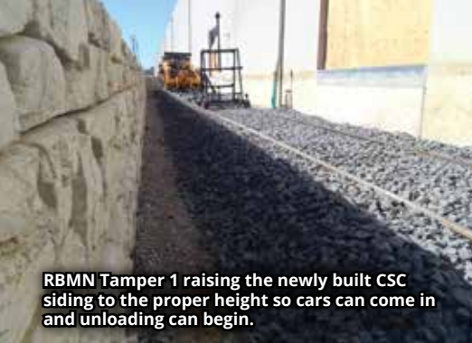
The RBMN tamper 1 in operation, tamping freshly dumped stone at the CSC siding.
