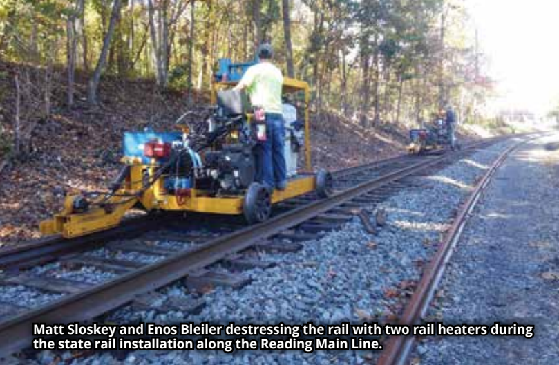
Multiple crews from the Reading MOW division installing a 1600' rail along the Main Line.
