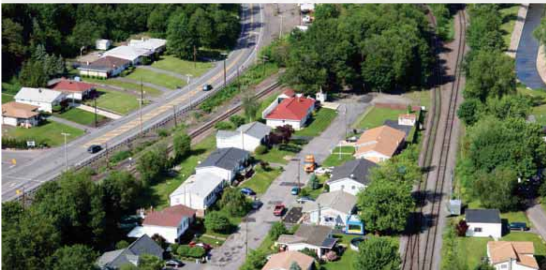
Aerial photo of the existing Dupont Interlocking. The track to the left is Canadian Pacific. The center of the photo is the connection track with CP as well as the crossover on RBMN. To the north of this crossover, a new switch will be installed.
