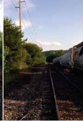
MP 87 on the Reading Mainline recently gauged to 56 1/2 inches after the 2013 tie work.
