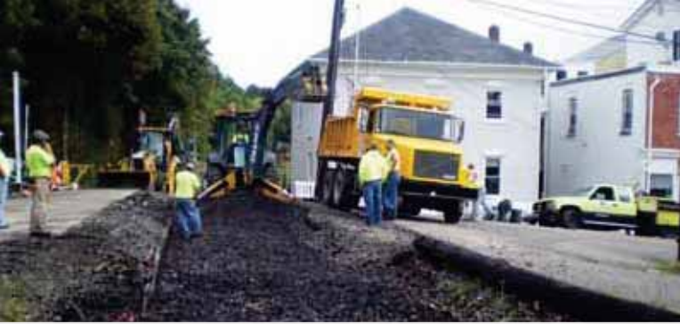
Track gang in process of replacing the Rt. 940 grade crossing in White Haven, September 2009 and their finished product.
