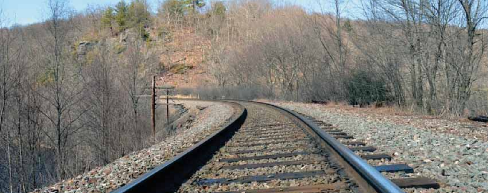
Curve on our mainline MP 135.3 where we replaced 712 ties, gaged, and surfaced it in 2013.
