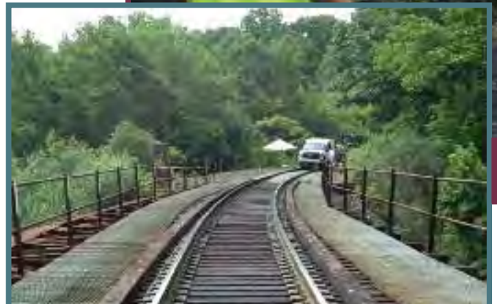
North end of Bridge 144.92 showing the brand new timber decking.
