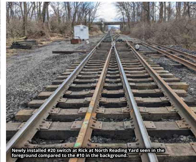
Newly installed timbers are spiked at the switch upgrade at Rick to #20 is completed by Tim L'Amie, Dave Hutton, Chuckie Carl, Dennis Rosohac, Tyler Acker, and Enos Bleiler.
