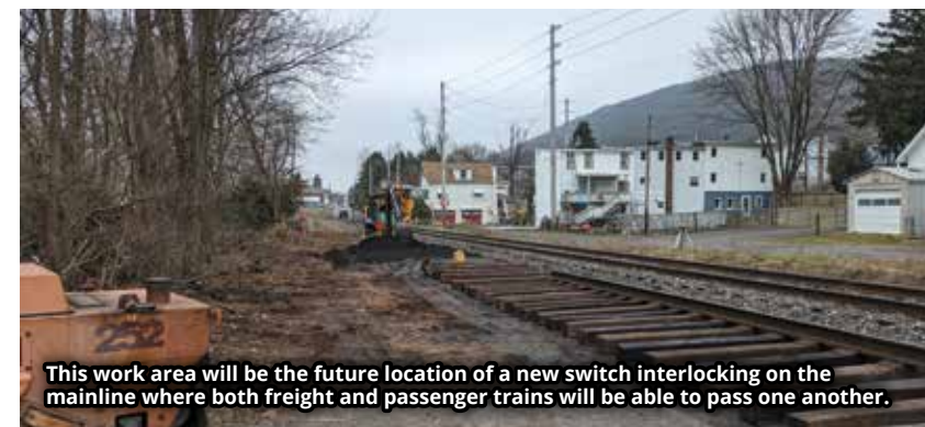
At the Nesquehoning Campus, a new main track is being built on the left side of the picture. The new track will join the original main track just north of this location.
