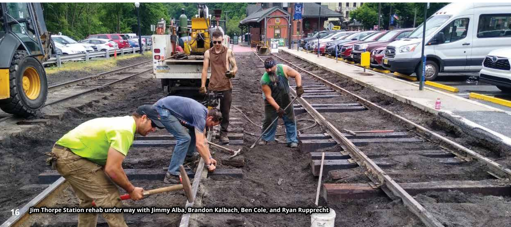
Railworks tie installation at M&S Branch MP 128.5.
