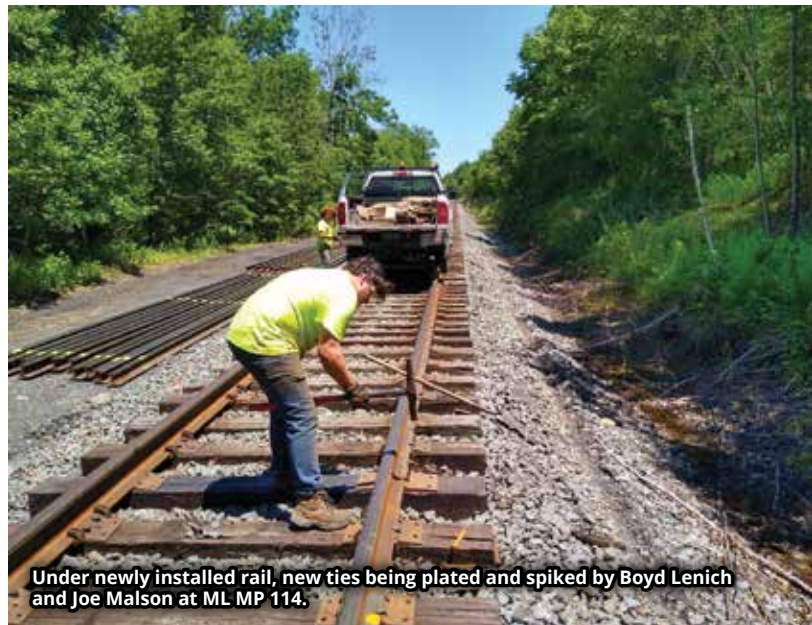
New rail being anchored by Chucky Carl, Ron Collins, Boyd Lenich, Joe Malson at ML MP 114.2.
