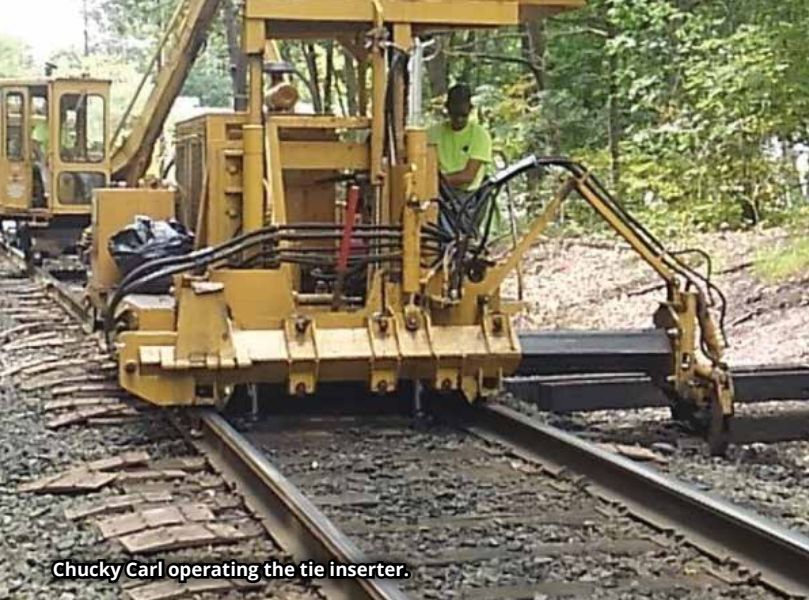
The Reading and Northern "Tie Gang" installing ties at East Mahanoy Junction.
