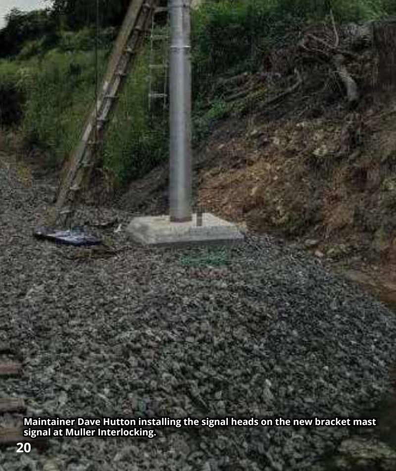
Maintainer Dave Hutton and Maintainer John Washburn were working to install the ladder to the newly installed bracket mast signal at Muller Interlocking. While Maintainer Darnell Young worked from above, install the railing to the upper platform from the bucket of BT-2.
