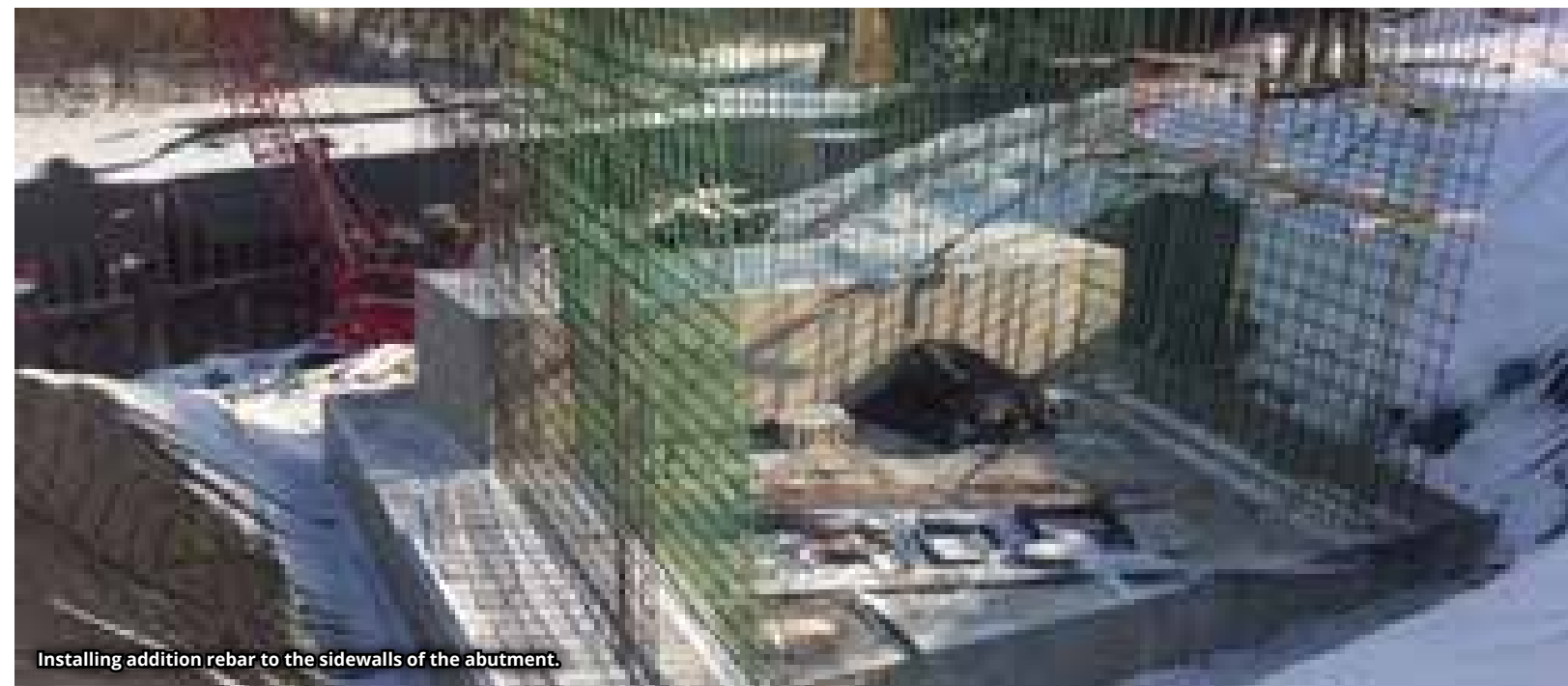
With the framing completed the next step installing rebar.
