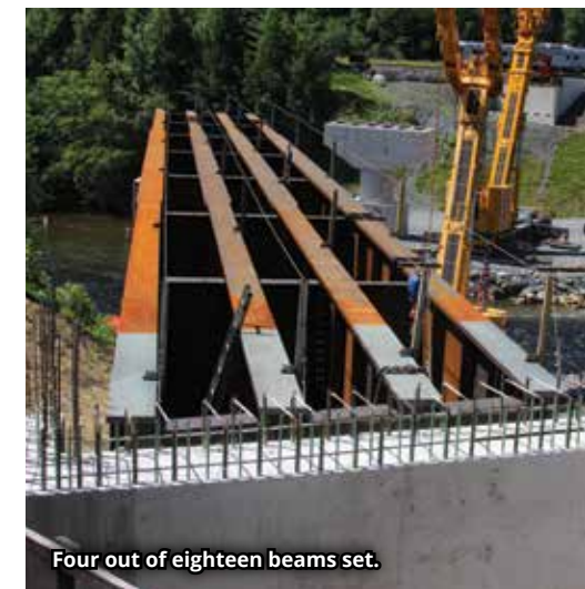
The second crane picking the beam from the center span and moving the one hundred, twenty-foot-long beam into place between abutment two and pier two.
