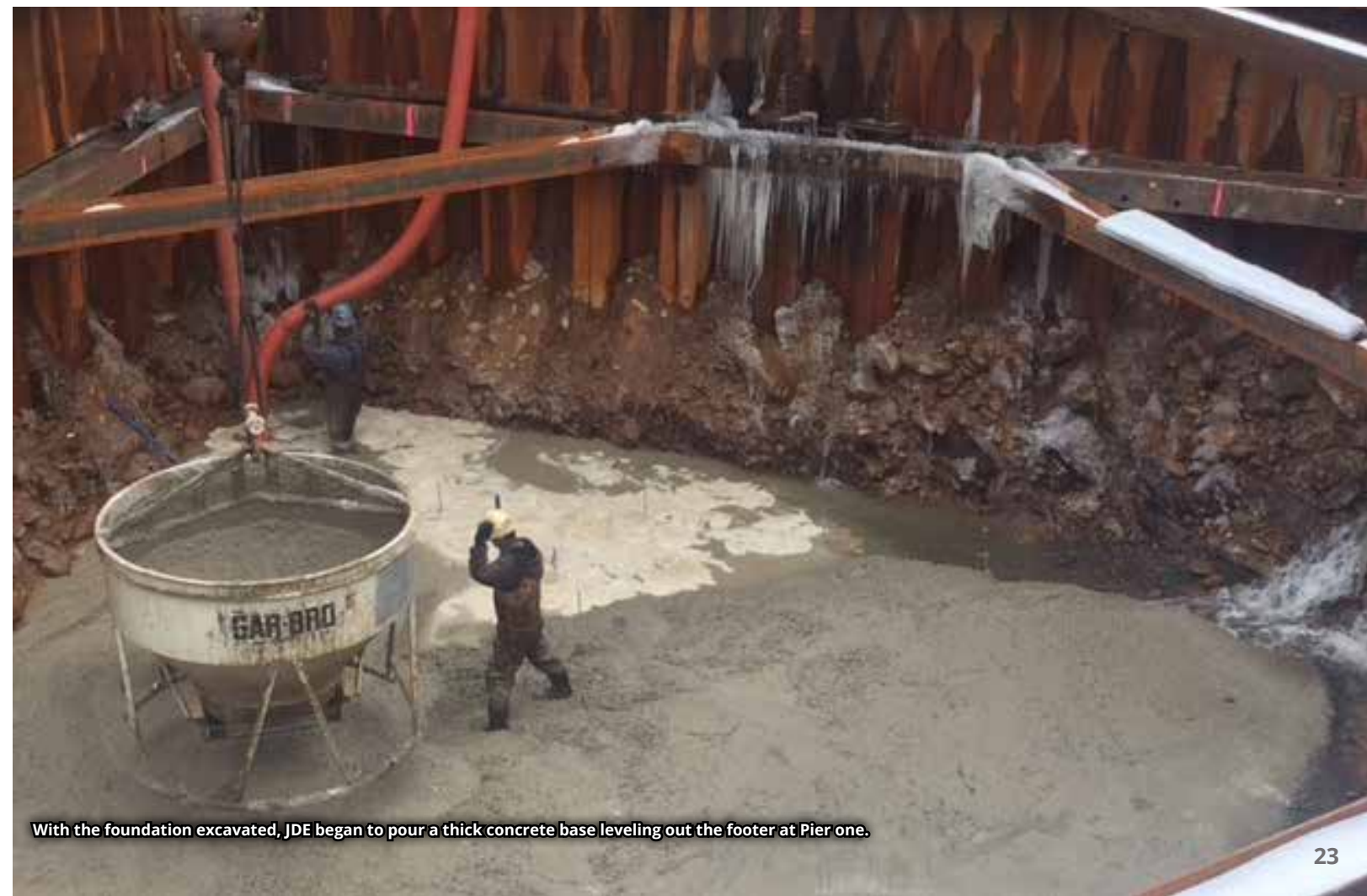
JDE constantly battled high water as they excavated out for pier one.
