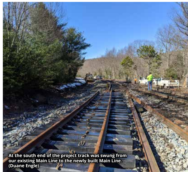
With the east rail in place, proceeding to install the west rail. From left to right (John Brown, Matt Sloskey, Alex Scubelek in backhoe, Charles Carl, Dennis Roshac, Duane Engle, Shawn Himmelberger in backhoe)
