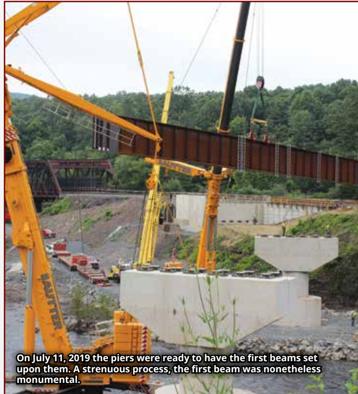
The first beam is finally set on the east side abutment and pier.
