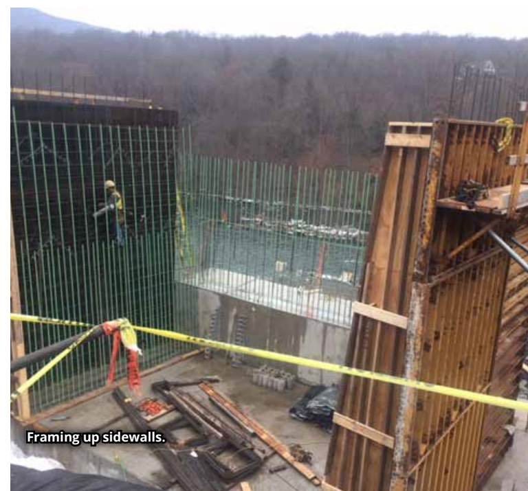
Installing addition rebar to the sidewalls of the abutment.
