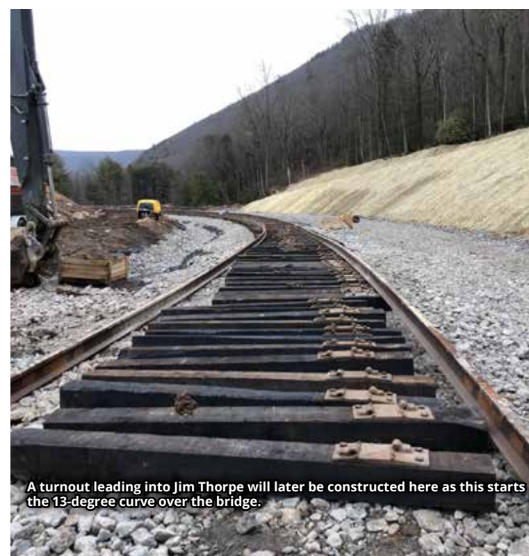
Rails were laid onto the bridge as they began track construction.
