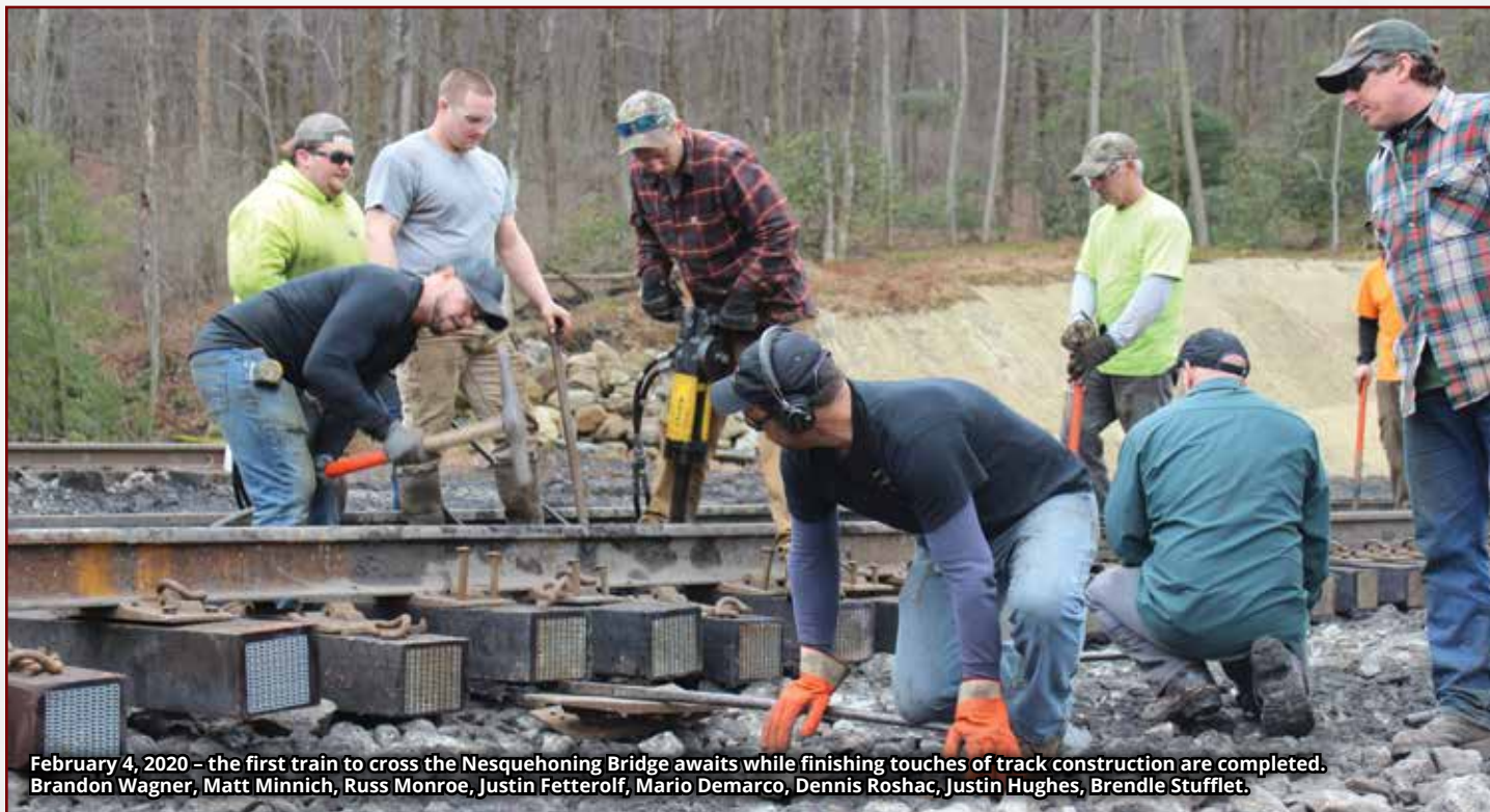
The track configuration leading to the Nesquehoning bridge required moving the main line. Ties are laid out in preparation of final track construction.
