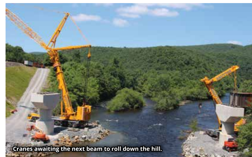
As the first beam makes its way down the hill a crane is positioned to pick and set each beam.
