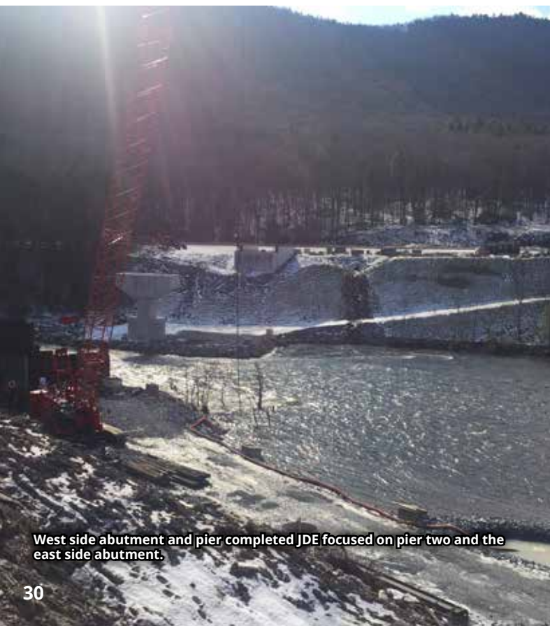
A crane was used to assist with setting forms for the pier.
