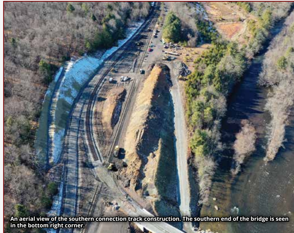
The track configuration leading to the Nesquehoning bridge required moving the main line. Ties are laid out in preparation of final track construction.
