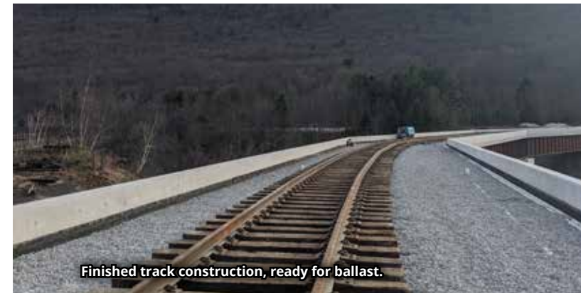
The new track leading up to and over the Nesquehoning Bridge would take over 1000 tons of ballast.
