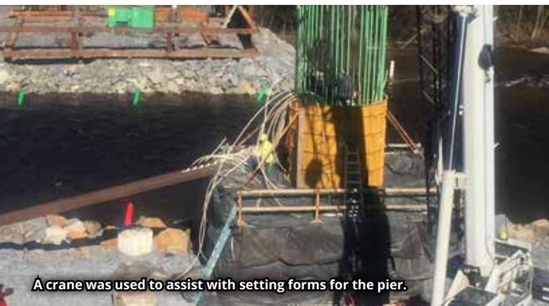
JDE working at the east side abutment and pier two.
