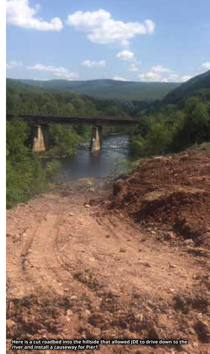
Contractor creating access road to project for causeway and abutment on east side.
