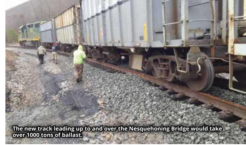
RBMN workers at the south end of the project work to disconnect our existing main line track to the left, shift the track and reconnect to the newly built track on the right.
