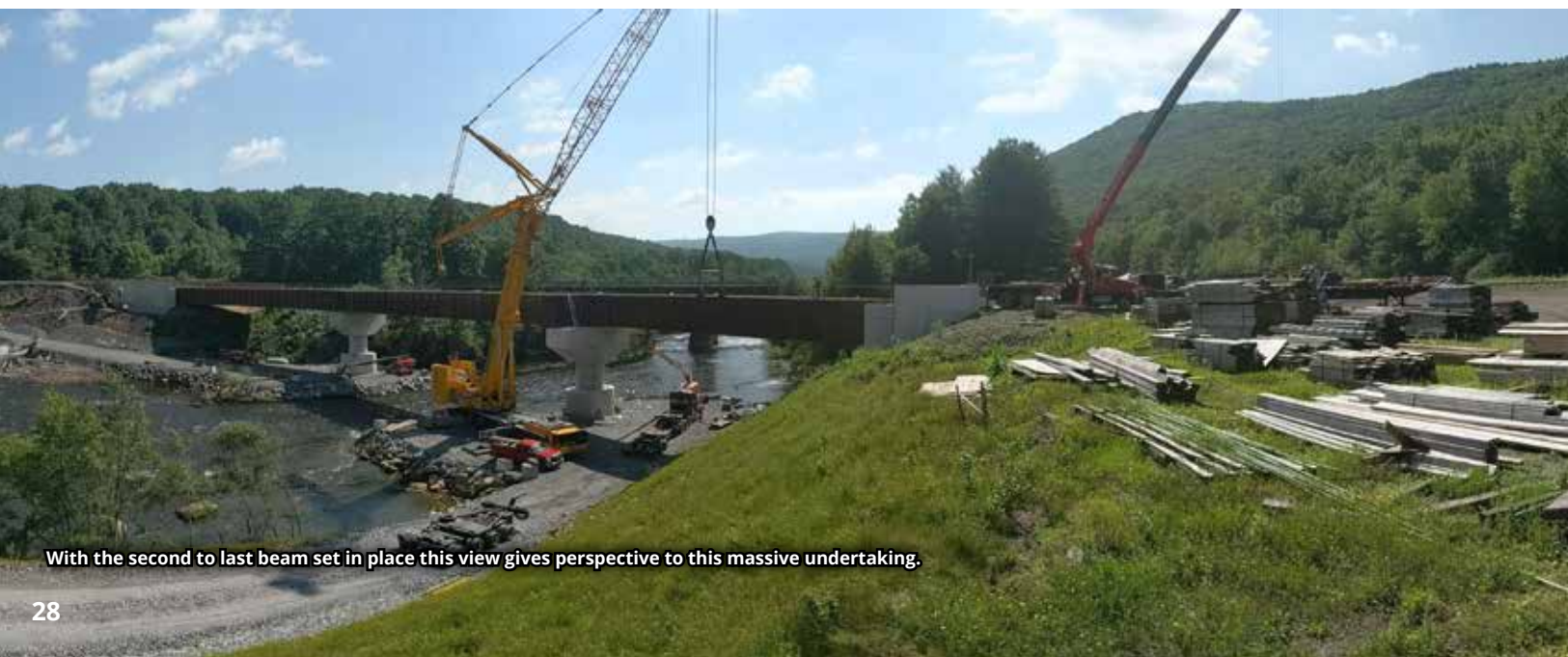
One of the massive cranes in position to lift beams.
