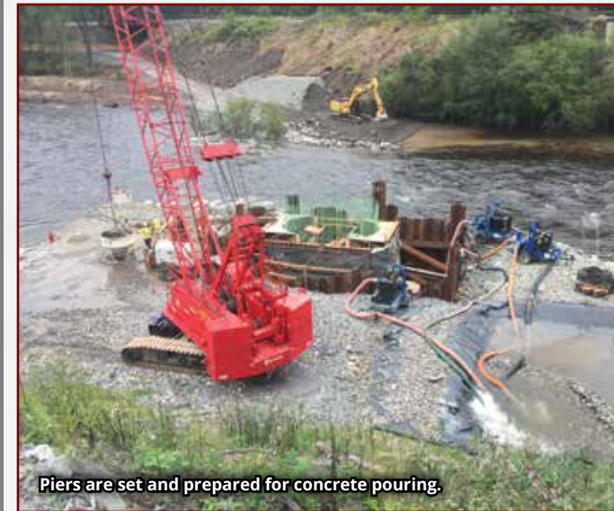
Piers are set and prepared for concrete pouring.
