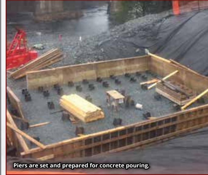
Piers are set and prepared for concrete pouring.
