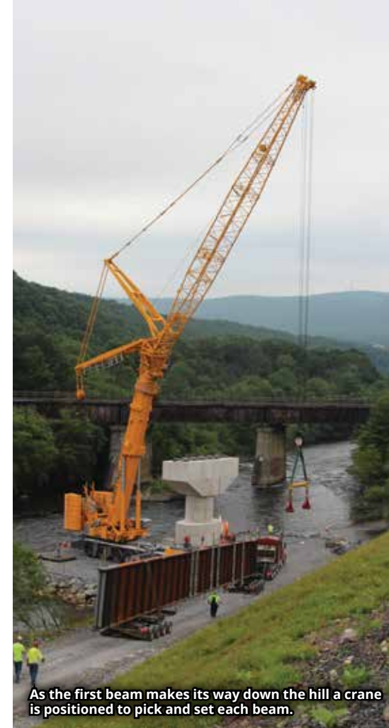
The second crane picking the beam from the center span and moving the one hundred, twenty-foot-long beam into place between abutment two and pier two.
