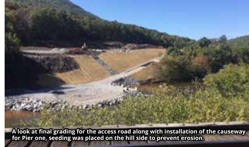
Upon removal of the brush and trees that were chipped into trucks and hauled away, JDE began to level and grade the new location for our Main Line.
