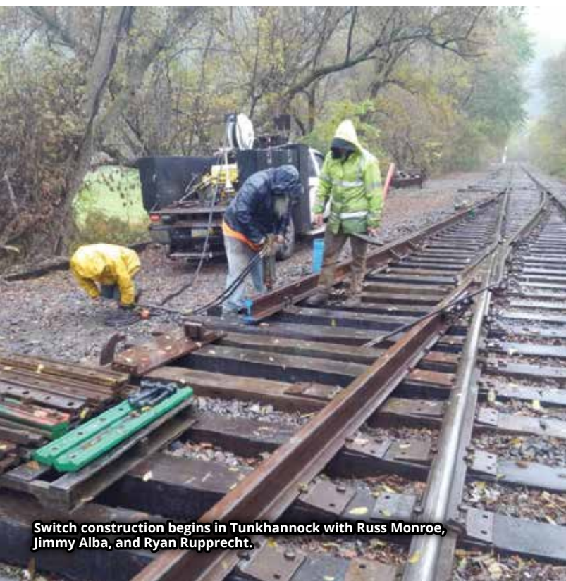
First ties, plates, and spikes get laid out for track one in Tunkhannock.
