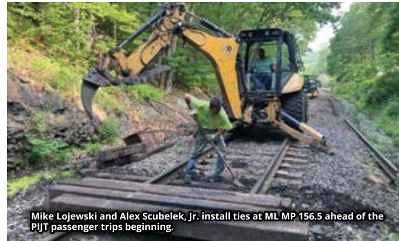
Mike Lojewski and Alex Scubelek, Jr. install ties during some work being done on the Pittston Wye for passenger moves.
