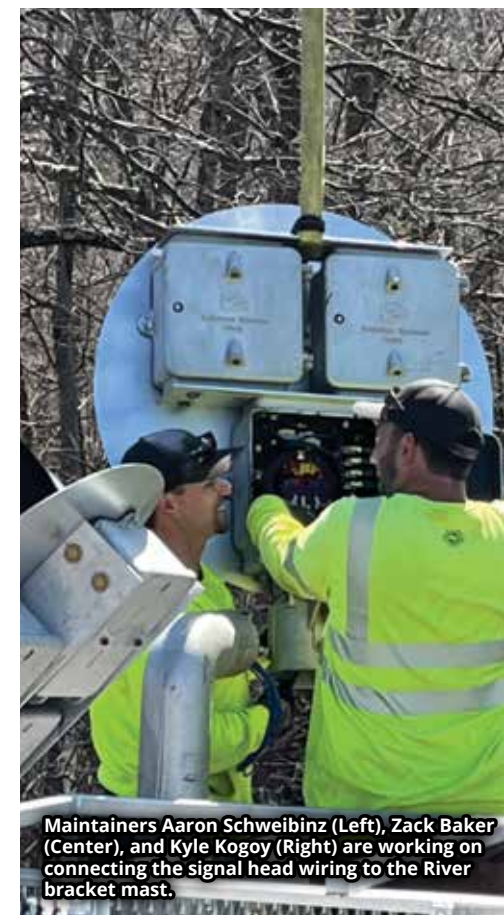
Maintainer Zack Baker working to align the signal heads at Nesquehoning Junction Interlocking.
