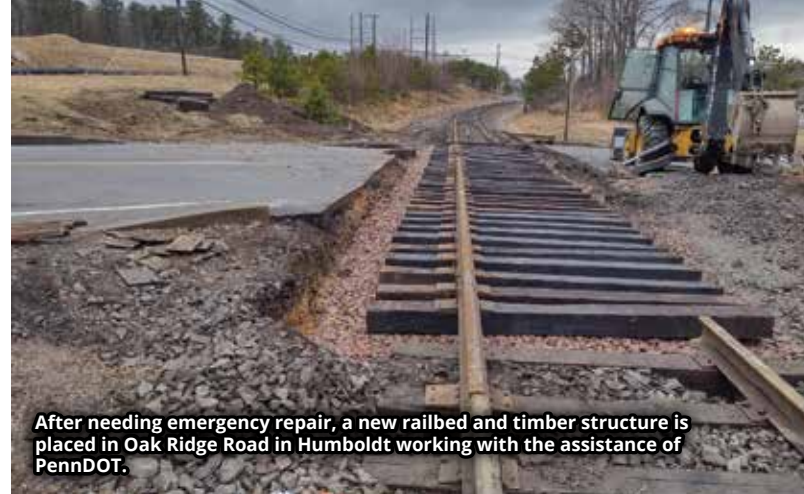
With new timbers, rail, plates, and OTM to fit, B. Kalbach and D. Hutton spike the plates down ahead of surfacing at Commerce Drive in Humboldt where PennDOT's 424 extension will soon enter the park.
