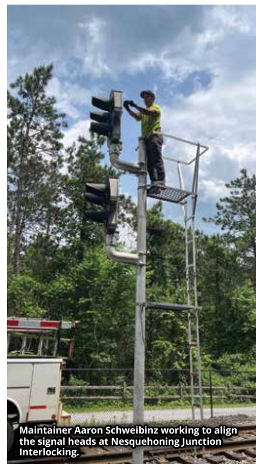
Maintainers Zack Baker (Left) and Aaron Schweibinz (Right) install signal heads on the River bracket mast before it is lifted into place.
