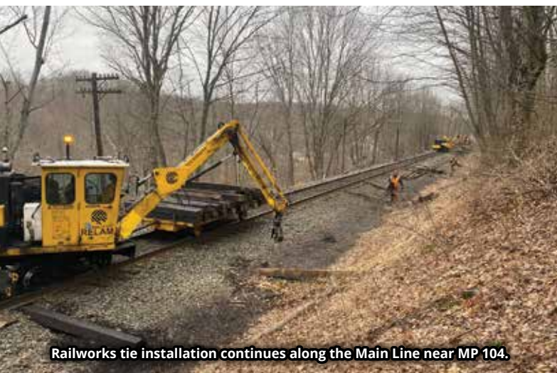
Railwork's machines are staged and ready to kick off the 16,000 tie replacement project along the Main Line at MP 106 in early March.
