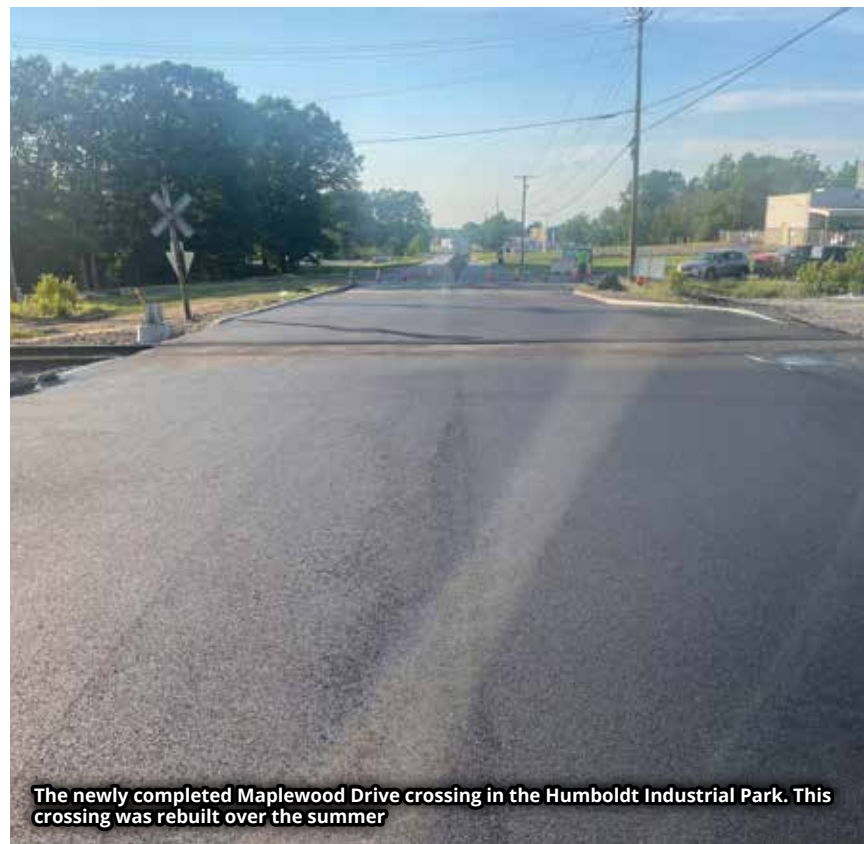
The Commerce Drive crossing is a new public crossing in the Humboldt Industrial Park. Once the roadway is opened, this crossing will allow the new extension of SR 424 to connect to the industrial park.
